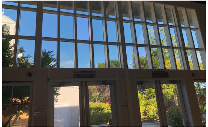
New windows in Findlay Hall.
