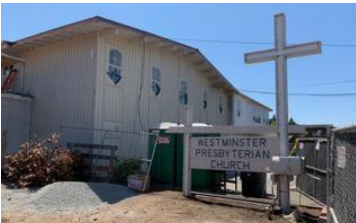
Awaiting new landscaping.
